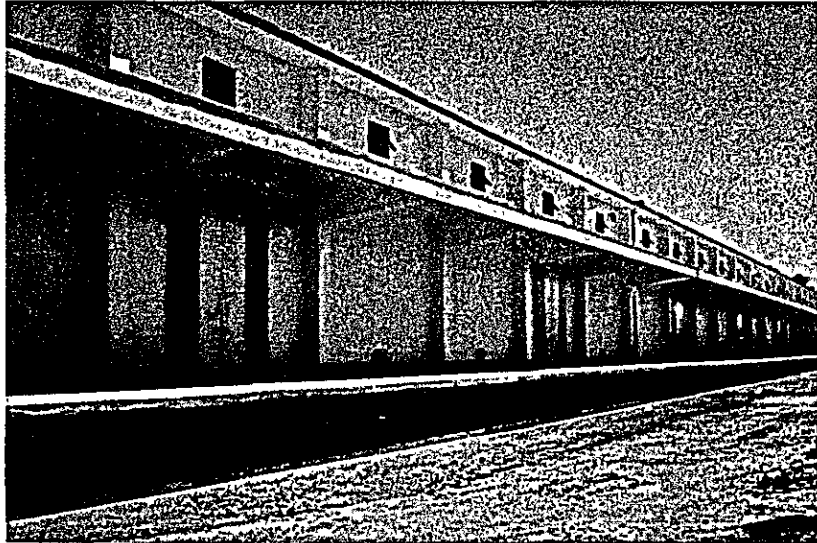
New Storehouses by the Japanese Grant of 1977 Capacity: 1,000 tons Maheswarpasha CSD, Khulna
