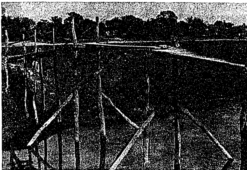
A bridge at Jinjira district
