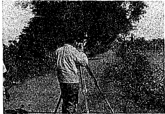
Establishment of Control Point
