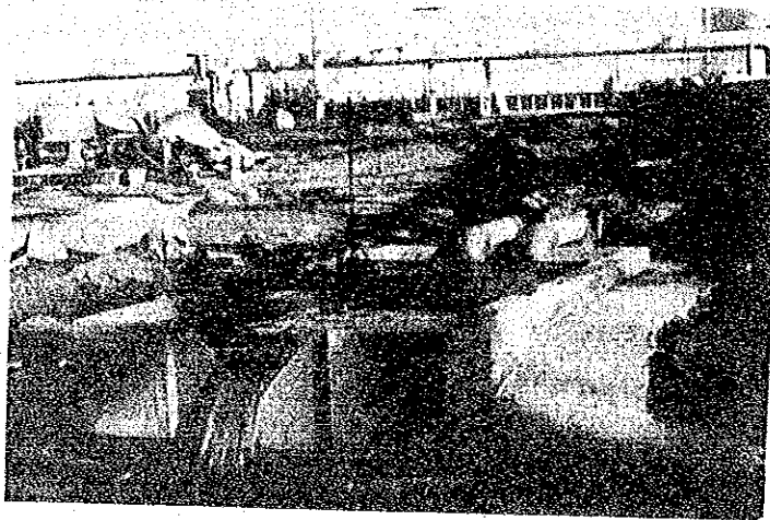
Photo 11: Water-gauging tank for measuring the flow (discharge)
