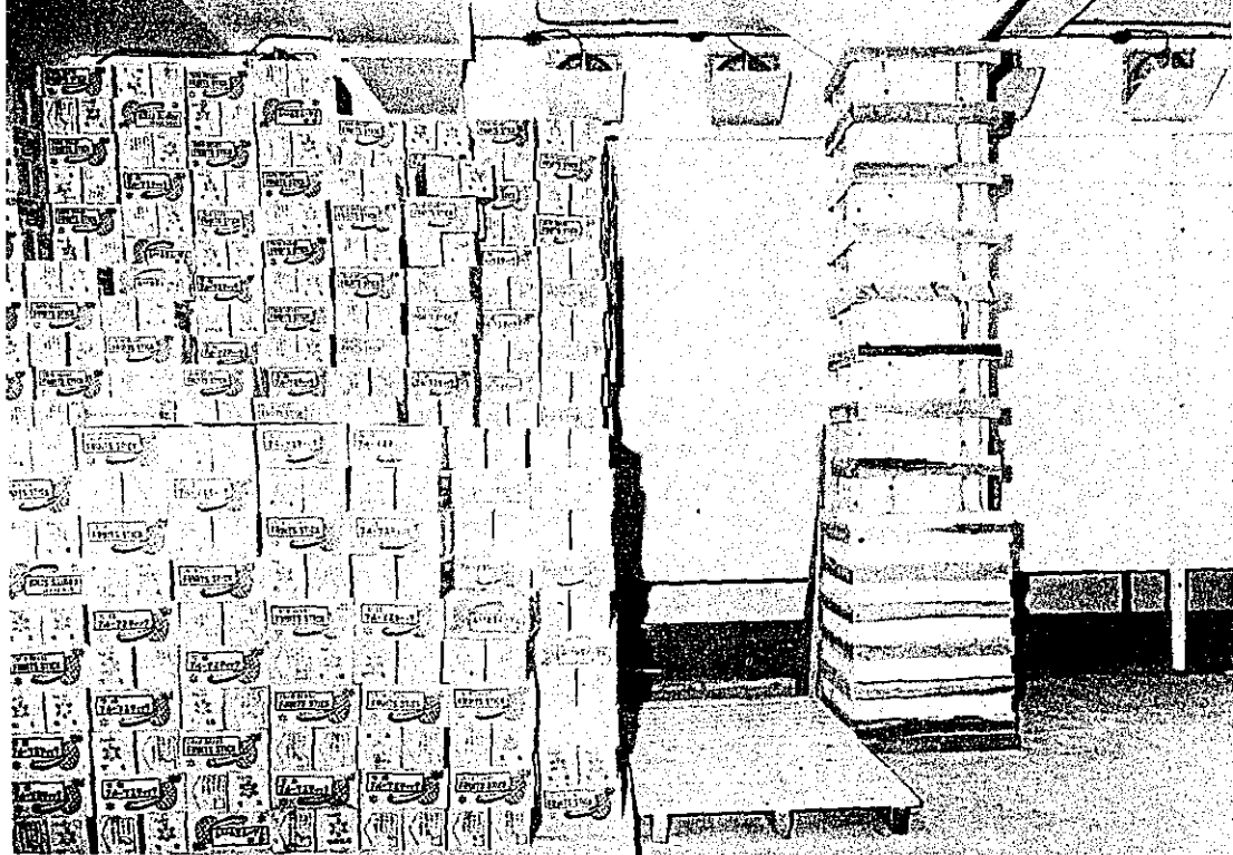
New type cold-storage room (air-blast system)
