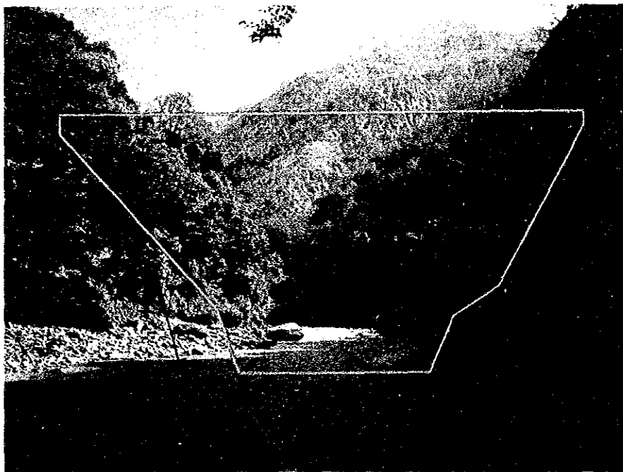
Arun 3 Dam Site — View from Downstream —
