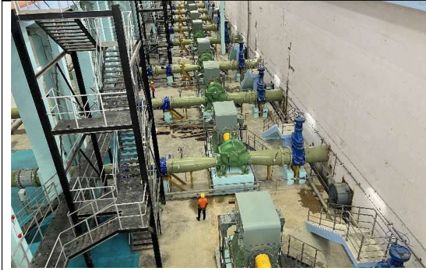
Site Visit at WTPs
