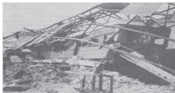
Plate.1. Railway station after the cyclone (November 24, 1978 by Rajah Studio, Batticaloa).
