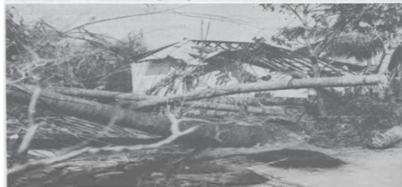
Plate.2. Cyclone damage on coconut plantations and houses (November 24, 1978 by Rajah Studio, Batticaloa)
