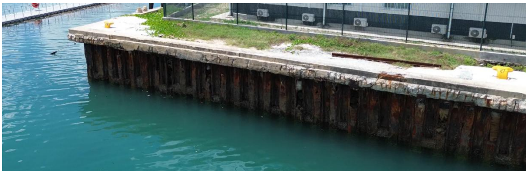
Figure 1-31 Corrosion condition of revetment steel sheet piles (installation location of mooring bollards northeast of the liquid bulk berth)
