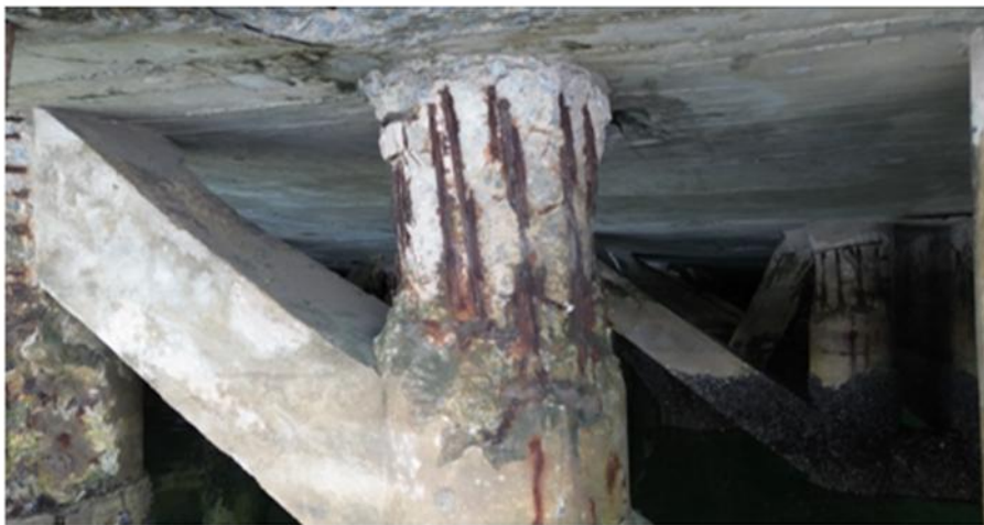
Figure 1-34 Progress of deterioration in the South Pier quay structure
