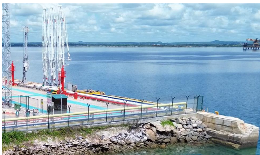
Figure 1-28 Liquid Bulk Berth, Loading Arms, and Fire Fighting Equipment
