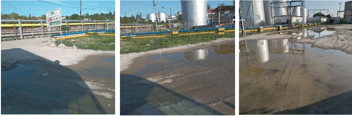
Figure 1-32 Water pooling near the vegetable oil tank
