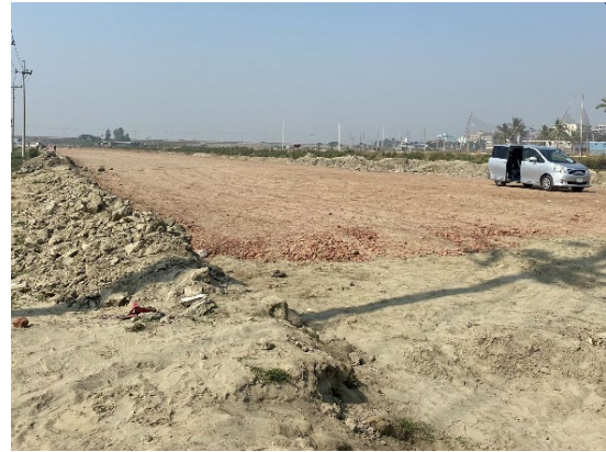
No.8 CDA Road (建設中)
