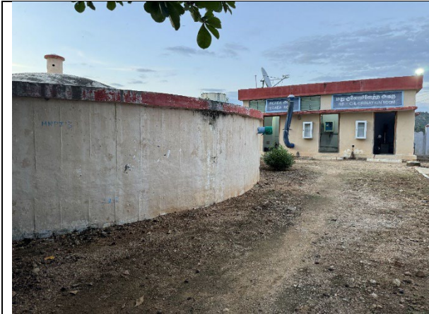
The SCADA Control Office, chlorine-injection facilities, and water distribution pumps are installed together.
