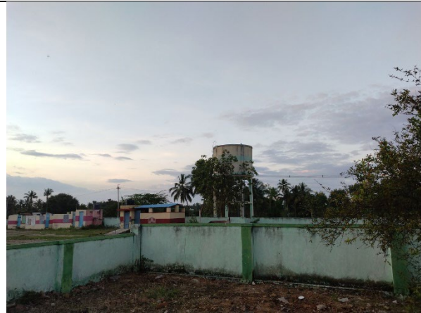
The OHT near the Union SUMP.
