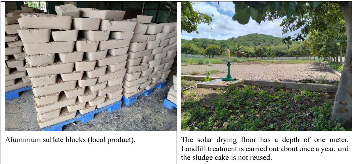
Figure 3.2.9 Present Condition of the WTP
