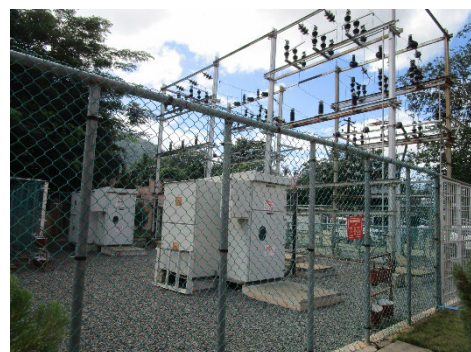
Figure 3.2.19 Outdoor 33 kV Power Receiving Facilities
