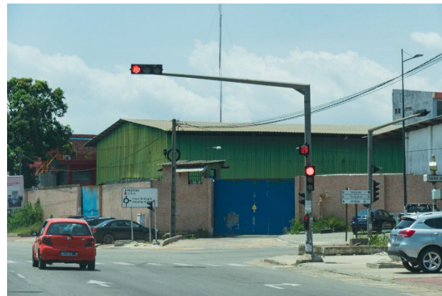
Traffic signals installed on major roads
