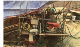
Drilling in dam site (angled)
