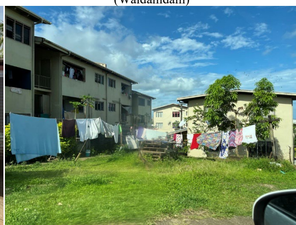
Public Housing Build in the Jittu Area
