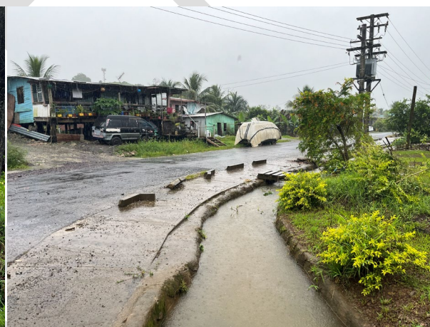
Drainage Improvement Conducted (Waidamdham)
