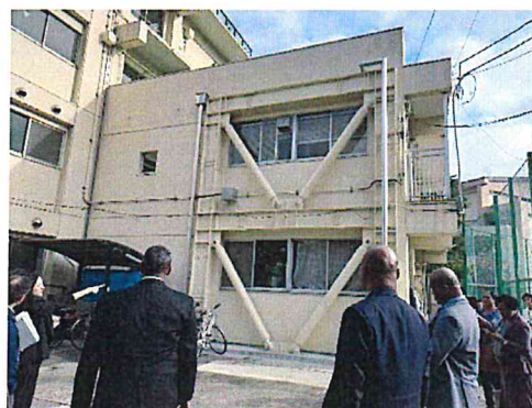
Fig. 14 Site Visit to a Seismic Reinforced School (Komadome Junior High School)
