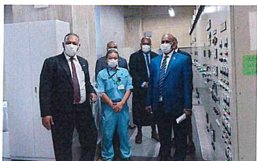
Fig. 13 Site Visit to Generator Room in Japan Red Cross Medical Center
