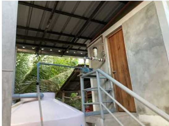
(Left) Electric pumps installed by residents at a rainwater-based water supply facility
