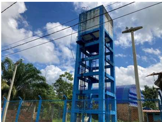
(Left) Elevated water distribution reservoir (water supply facility that pumps up groundwater)
