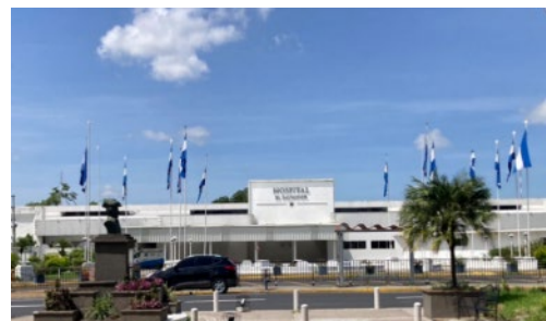
Front view of Hospital El Salvador (photo by the evaluator)
