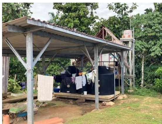
Rainwater-based water supply facility 1
