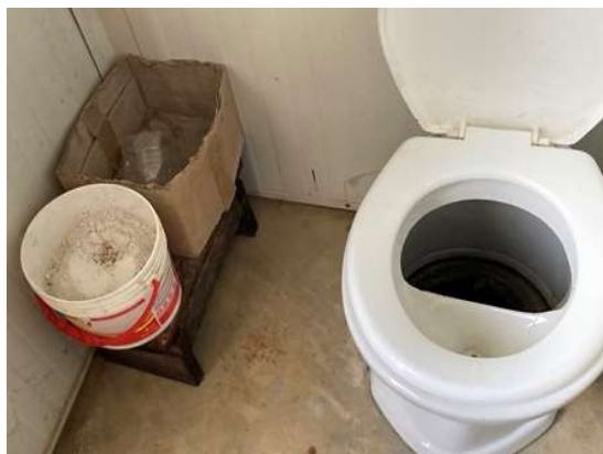
(Left) Composting toilets (separate urinal and feces), material for drying (ash and sawdust)
