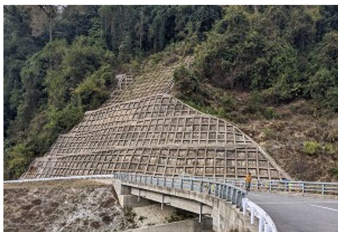
Slope Protection Works at Beteni Bridge (Source: Photo taken by the evaluator)
