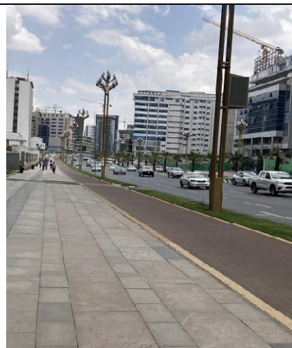
Road after Completion of the Corridor Project
