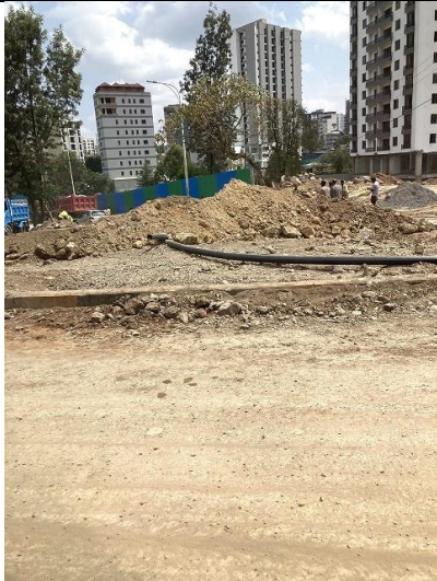
Excavated Area of the Corridor Project (Exposed Pipes)
