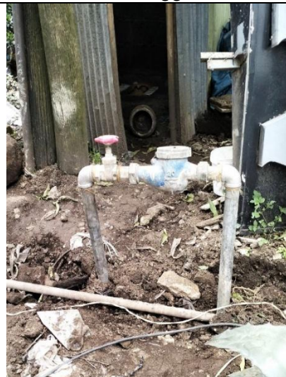
Customer Meter after Installation Correction Photo Provided by Mekanisa Branch
