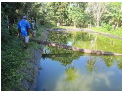
Figure 24 Damaged community ponds
