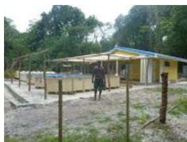
Completed Mangaliliu Community Sea Farming Centre
