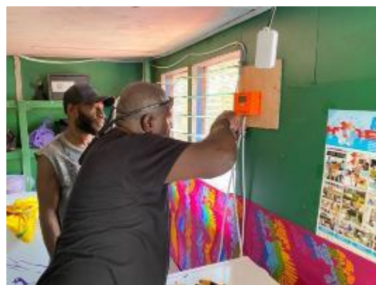
Installation of solar freezers
