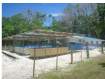
Mangaliliu Community Sea-farming Centre, where renovation work has been completed after Cyclone Harold
