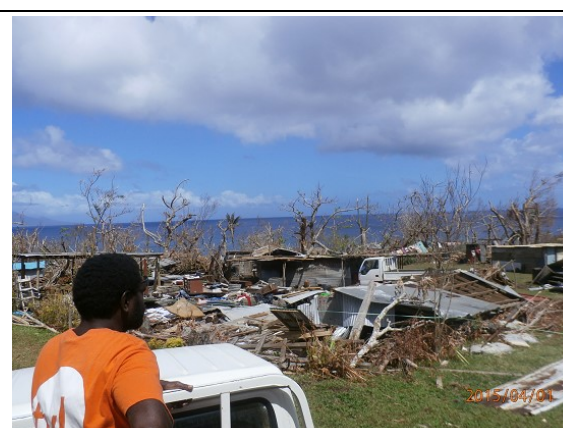
Photo: Houses destroyed by strong wind of the Cyclone (Malalip, Efate Island, Shefa
