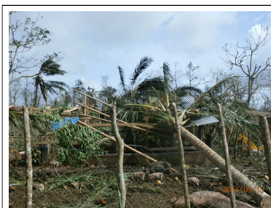
Photo: Coconut trees collapsed on livestock breeding facility (Teoma, Efate Island,
