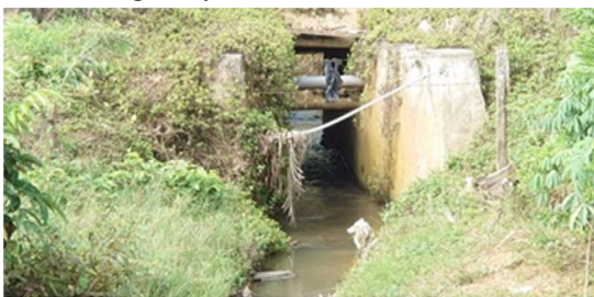
Source: JICA Consultant Team, Sep.2022
