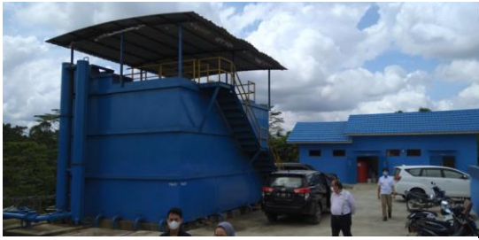
Source: JICA Consultant Team, Sep.2022
