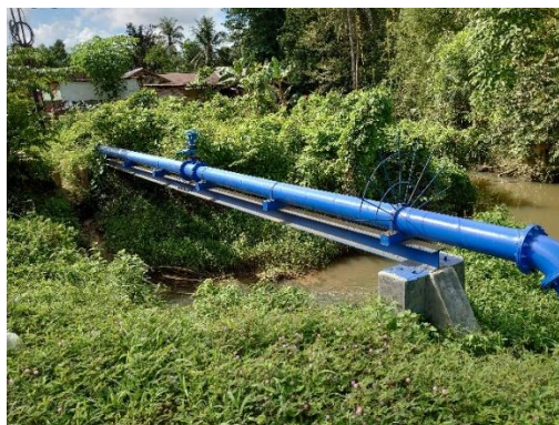
Figure 5-36: Water Pipe Bridge Crossing Drainage Canal
