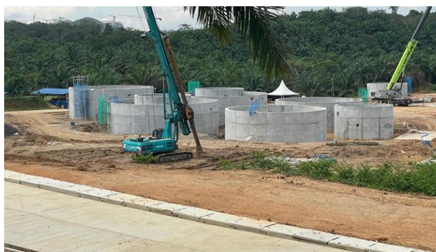
Source: JICA Consultant Team (02 MAY 2024) Figure 5-31: Construction Site of WWTP 1
