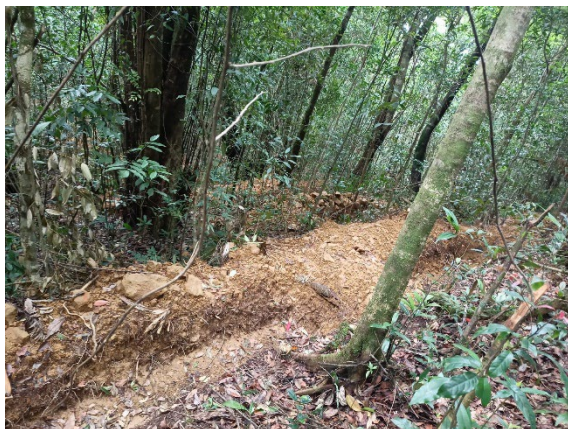
A Staggered Trench in Ailawng by Land Resources Department, Mizoram (source: JICA Survey team)
