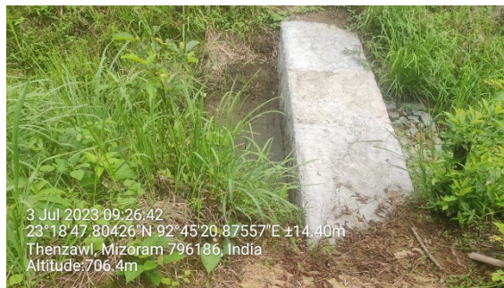
RR stone masonry Gully plugging in Thenzawl north village (Source: JICA Survey Team)
