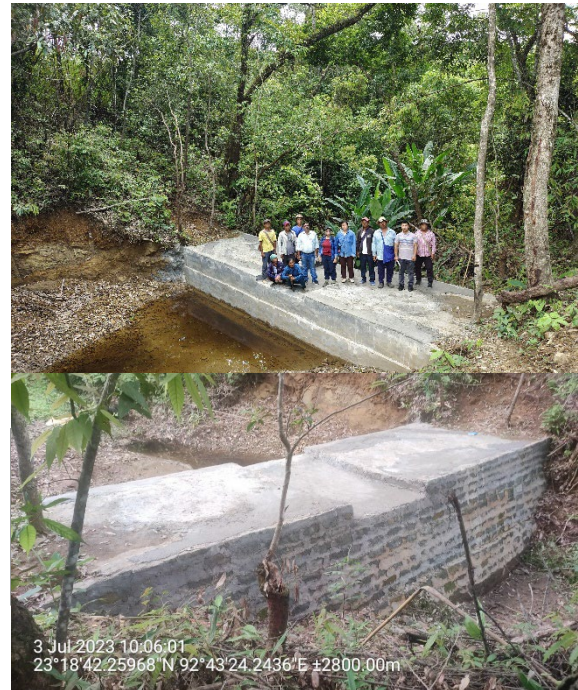
D/S photo of RR Stone masonry check dam (Source: JICA Survey Team)
