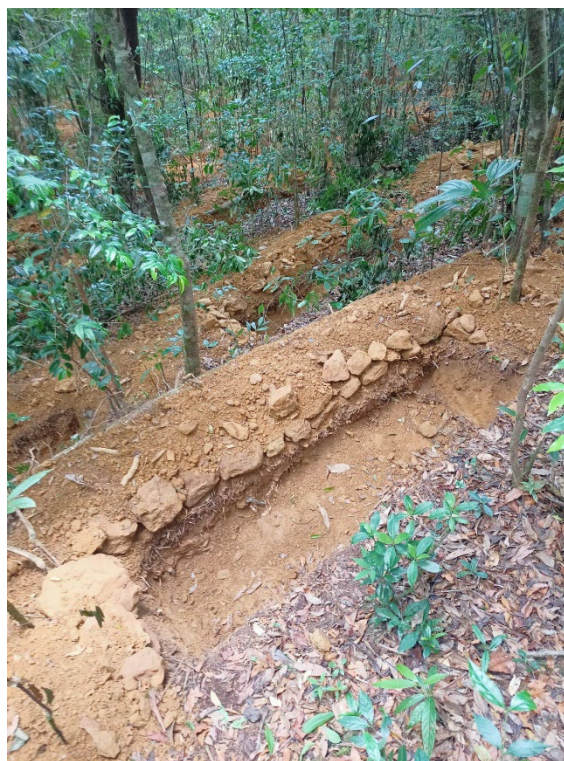
A Staggered Contour Trench in Ailawng by Land Resources Department, Mizoram (Source: JICA Survey Team)
