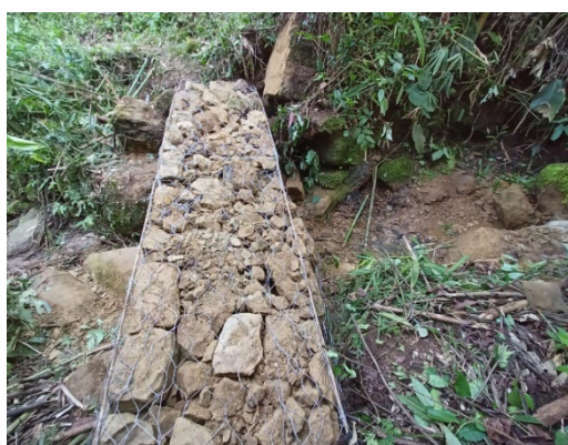
A Gabionic Check Dam in Ailawng supported by PMKSY-WDC 2.0 implemented by Department of land resources, Mizoram
