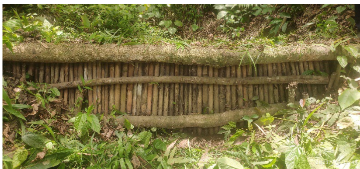
A Gully Control Structure using vegetative measures by using locally available materials such as dry wooden stumps, bamboo and loose boulder stones and mud in Thenzawl Forest Division, Mizoram (Source: JICA Survey team)
