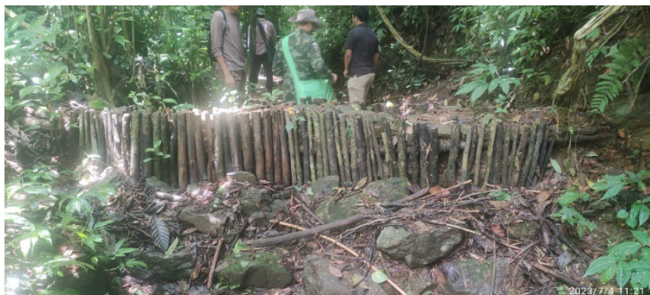
A Gully Control Structure using vegetative measures by using locally available materials such as dry wooden stumps, bamboo and loose boulder stones and mud in Lunglei Forest Division, Mizoram (source: JICA Survey team)
