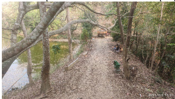
An Earthen Check Dam in Kawrthah Forest division, Mizoram (Source: JICA Survey Team)
