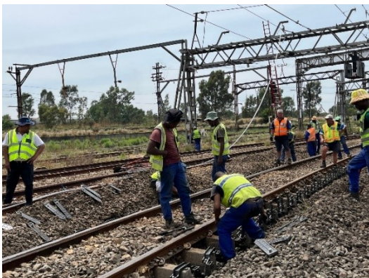
Installation of the sleeper anchors
