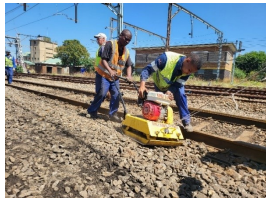
Grading after installation of the sleeper anchors
