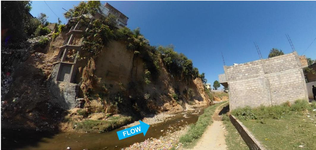
Cliffs are collapsing due to soil erosion caused by flood. (Upstream)
