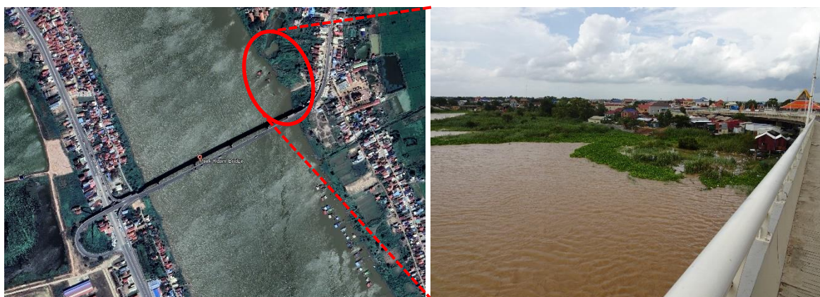
Figure 7.4-4 Condition of River Bank around Prek Kdam Bridge
