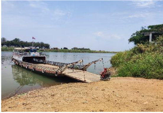
OD-1 Ferry port (NR1 side)
