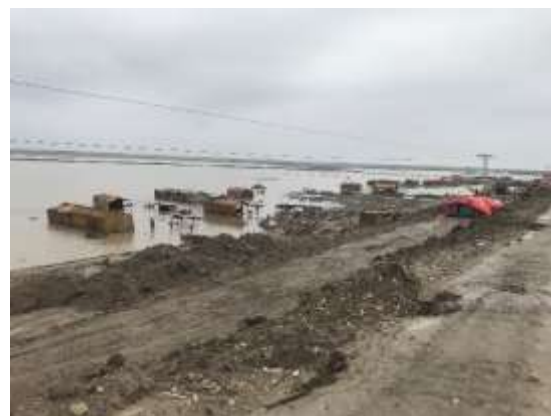
Photo 4.2.2 Situation of the landside of the MCB
