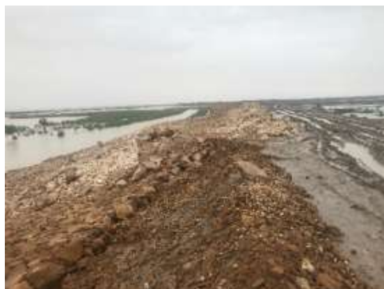
Photo 4.2.1 Situation of the top and lake side of the MCB
