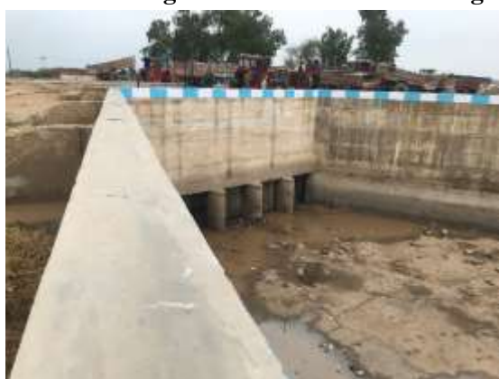
Photo 4.2.3 Situation of Danister Head Regulator(1)
