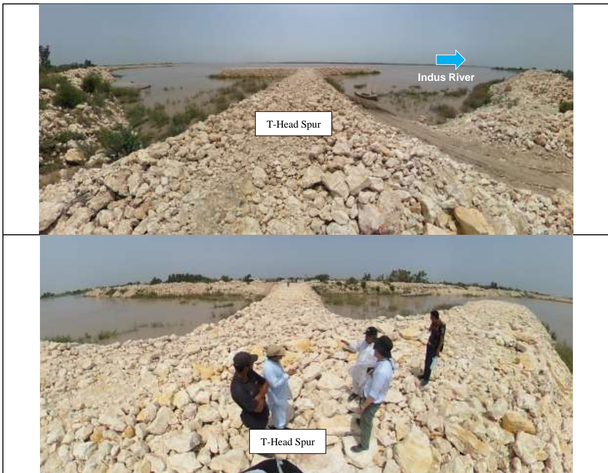
Photo 1.1.14 T-Head Spur at L.S. Bund, Hakra Point, August 4, 2023
