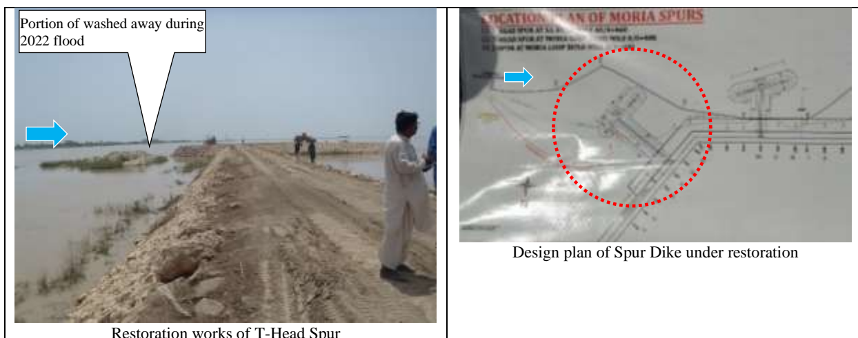
Photo 1.1.5 T-Head Spur Dike under restoration at Moria Loop Bund, August 3, 2023
