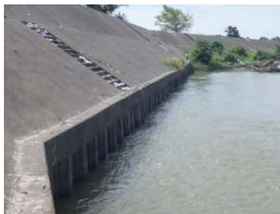
Photo 3.6.8 Sample of Sheet Pile Revetment in Front of a Bund (Philippines)
