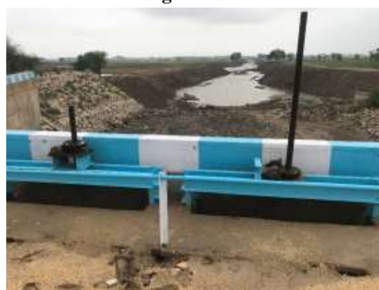
Photo 4.2.4 Situation of Danister Head Regulator (2)
