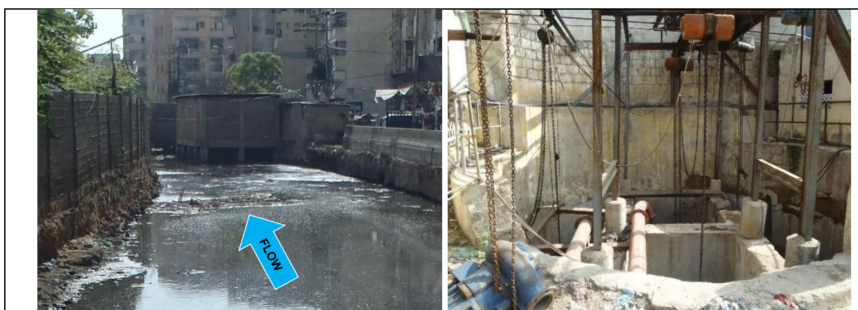
Drainage facilities in Karachi: (left) buildings constructed within drainage channel, (right) Pitcher drainage station, installed in 1993, aging and lacking drainage capacity
