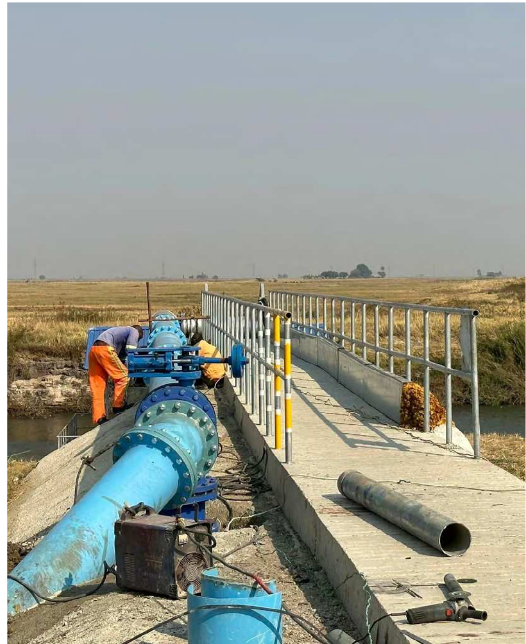
Maintenance works on the Rising main in WWSC
