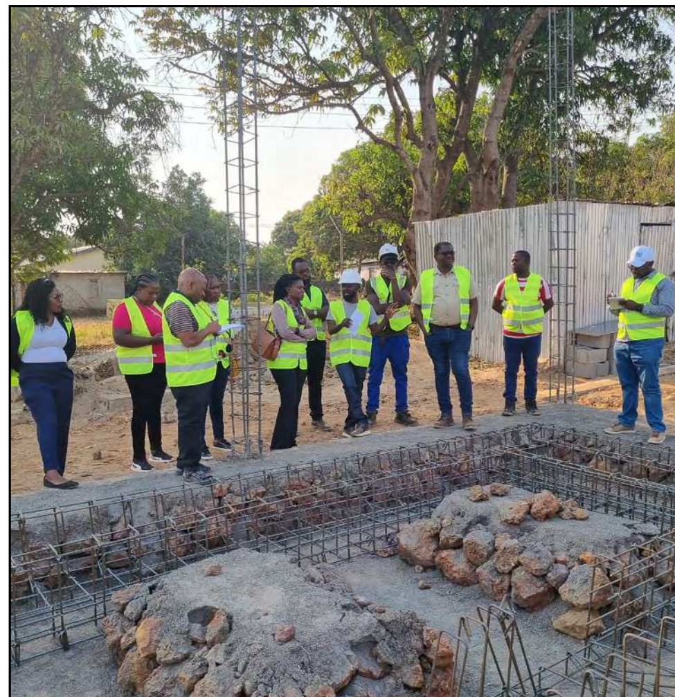
Construction of Water Infrastructure.
