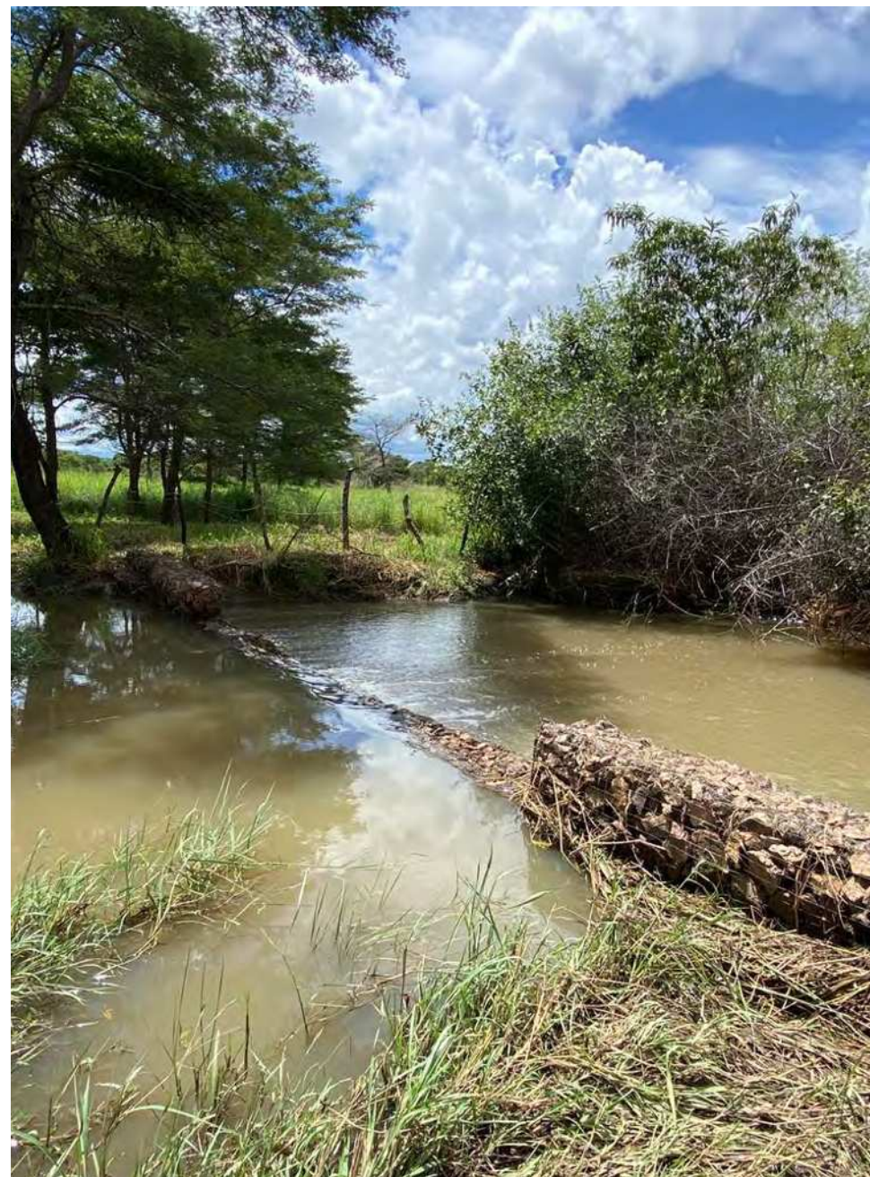
Mponda Check dam in Mumbwa
