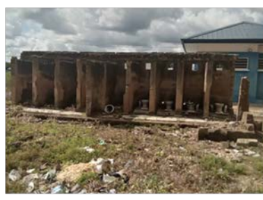
Abandoned "Toilet Area" for Travelers
