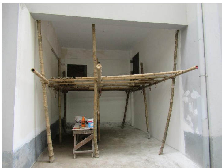
Pic. 27 Walls of PWD HQ buildings retrofitted with ferrocement
