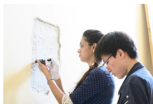
Pic.16 Application of a NDT method to a building in Dhaka
