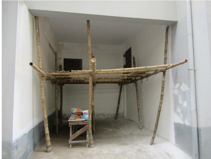
Pic. 27 Walls of PWD HQ buildings retrofitted with ferrocement
