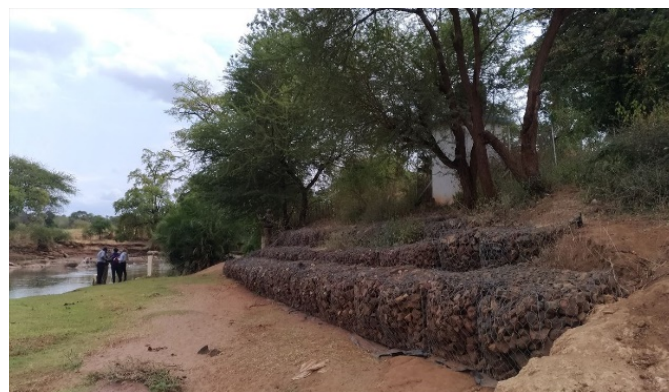
Candidate Gauging Station for Discharge Measurement Practices, 4F10 Kathita in Meru SBO. Gabion mattress installed in the Previous Advisory Activities. (2021/7/8)
