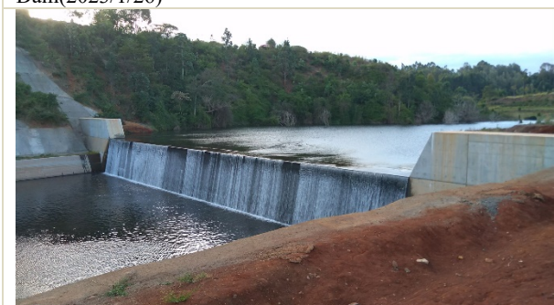
A Check Dam located at the upstream part of Thiba Dam (2023/1/26)
