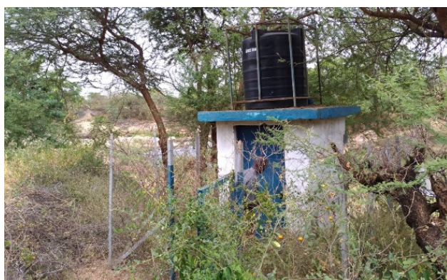
Candidate Gauging Station for Discharge Measurement Practices, 4F10 Kathita in Meru SBO. A small building for accommodating data logger system. (2021/7/8)
