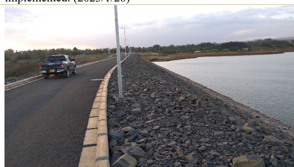
Thiba Dam Body looking from the left bank side. (2023/1/26)
