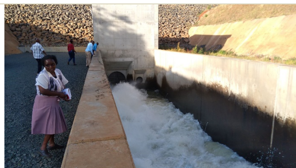
Irrigation Outlet of Thiba Dam. Flow Release of 5 m 3 /s implemented. (2023/1/26)
