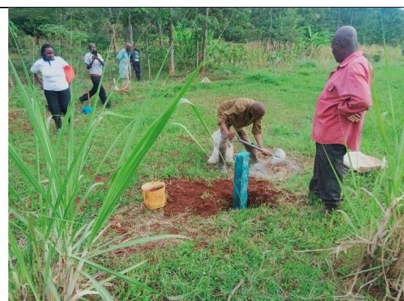
Riparian marking activities in the Muranga Sub-basin Office. Under the guidance of WRA staff, residents are installing concrete posts indicating the maximum water level during floods.
