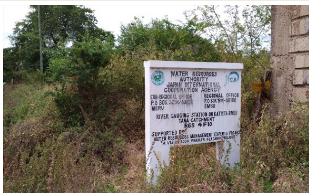
Candidate Gauging Station for Discharge Measurement Practices, 4F10 Kathita in Meru SBO. This Station was rehabilitated in the Previous Advisory Service. (2021/7/8)
