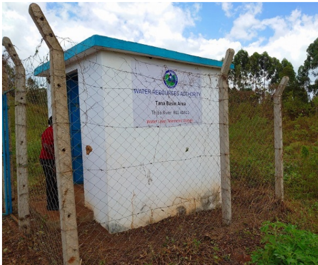
Site visit to Telemetering Station at 4DA11 Thiba. Outer view of the station building. (2021/10/26)
