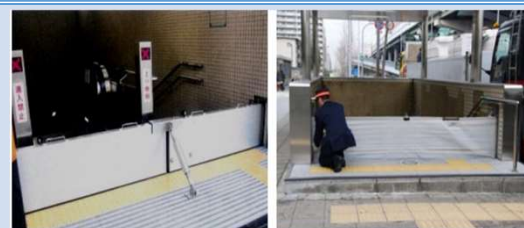
Water Shut-off Board at the Entrance
