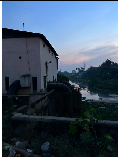
Bondajan Sluice Gate PS
