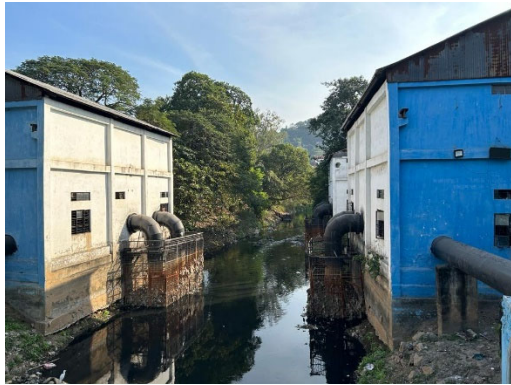
Bharalu Drain Pumping Station
