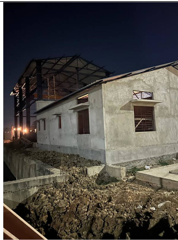
Under Construction Silsako Lake PS
