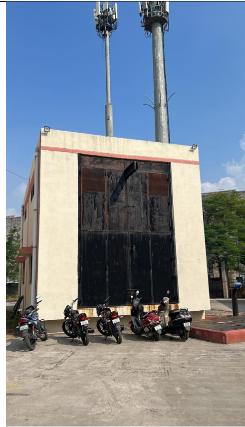
Veзалpur Storm Water PS of 5MLD Capacity (2W + 2S pumps configuration)
