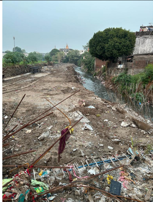
Koyli Creek Last Stretch Where Work Yet to Start
