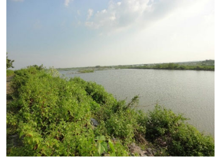
Area Where Land Acquisition has not been Completed in Jabung Regulating Reservoir (used as fishpond) (Source: external evaluator)
