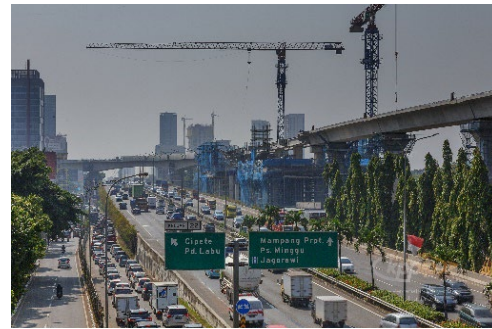
MRT North-South Line Project promoted by the project (under construction, August 2017)
