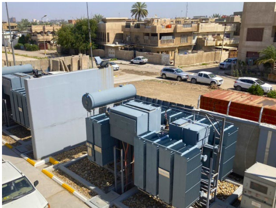
Newly constructed 33 kV substation (in Baghdad, left: transformer, right: control unit)
