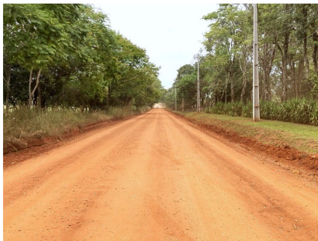
Gravel paved rural road 1
