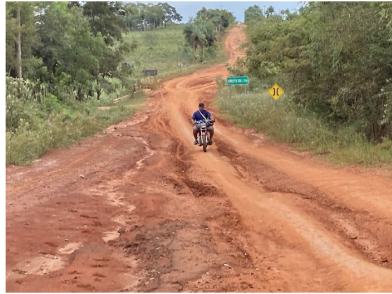
Example of unpaved road
