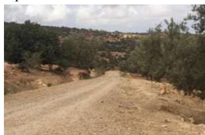
Rural road improved by the project (Source: taken by the evaluator)
