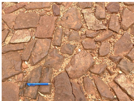
Surface of rubble paved road
