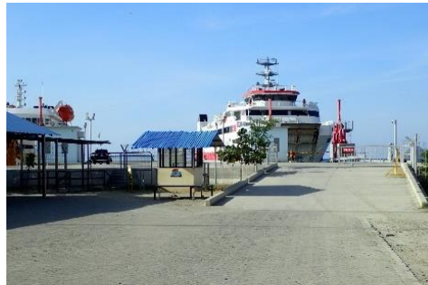
At the new ferry terminal (corridor to ferries) (source: evaluator)
