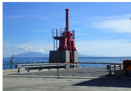
Movable ramp (source: evaluator)
