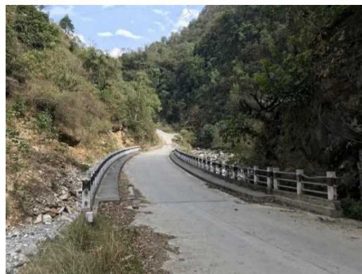
The Rangrung River Bridge Subject to Barhakilo-Barpak Road Bridge Project
