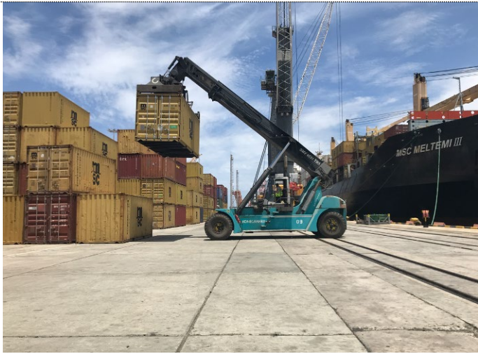
Concrete paved apron/yard (source: photographed by the evaluator)
