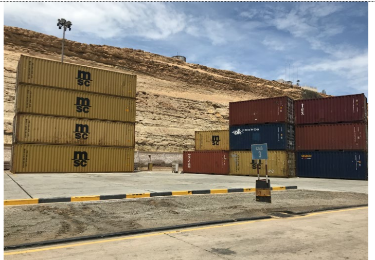
Concrete paved reefer container yard (source: photographed by the evaluator)
