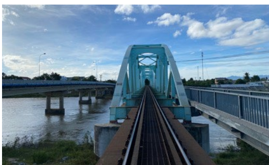
Image 2: Thap Cham Bridge and its side road in Ninh Thuan Province. The bridge used Japanese technology such as directly fastened track. (source: Photographed by the ex-post evaluator)
