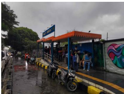
Bus Shelter in Kota Depok Developed Based on Pilot Project Findings (Source: Field survey)
