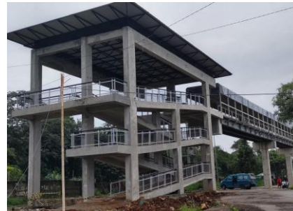
Improvement of Transportation Nodes in Kabupaten Bogor 3 (Source: Field survey)
