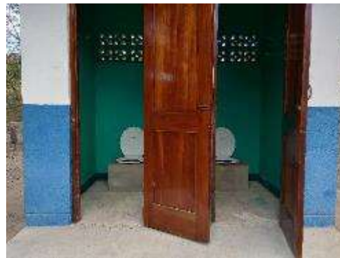
Photo 8. Toilet Booths Constructed by the Project (Nueva Segovia)
