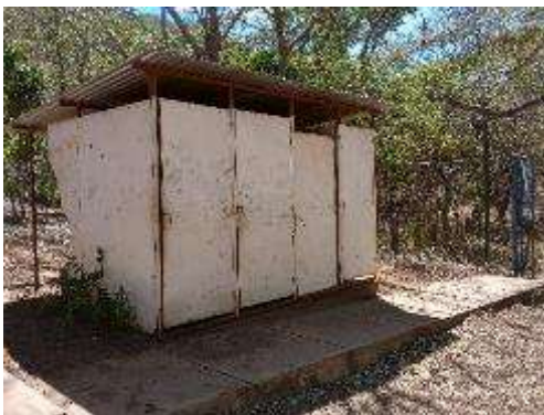
Photo 7. Toilet Booths which Used to be Utilized Before (Madriz)
