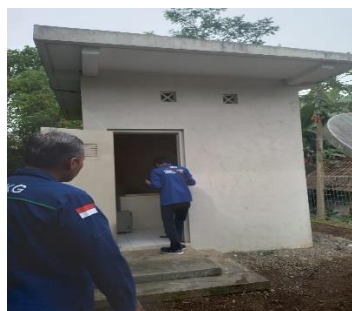
A seismic station constructed to install the seismic observation equipment
