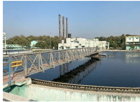
Sewage treatment plant constructed by the Project (Source: evaluator)
