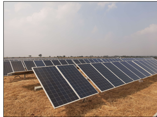
Solar power plant eligible for the project (Source: Evaluator)
