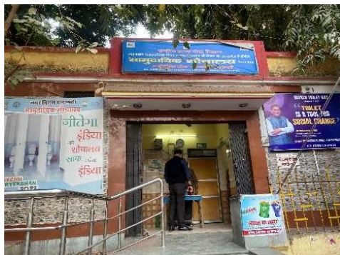
Community toilet constructed by the Project
