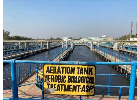
Aeration tank of the STP Source: Evaluator
