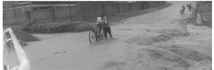
Figure 15.3.4 Poor Drainage Conditions due to Insufficient Flow Capacity of Drainage Infrastructure in Kampala Capital City
