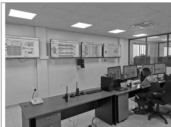
SCADA system in Katosi WTP (centralised management system)
