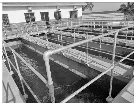
Rapid sand filter in Entebbe WTP
