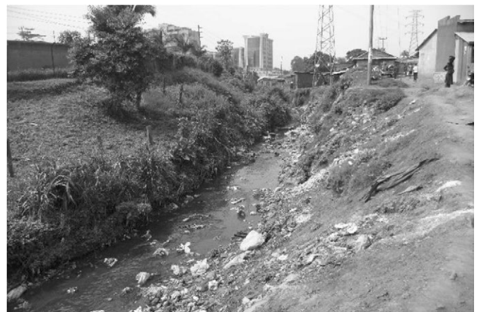
Figure 15.3.5 Collapse of Drainage Channel Slopes in Kampala Capital City
