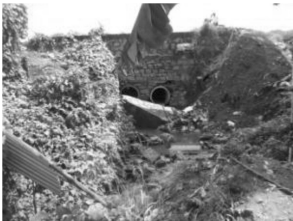
Figure 15.3.5 Collapse of Drainage Channel Slopes in Kampala Capital City
