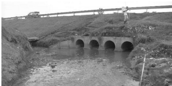
Figure 15.3.4 Poor Drainage Conditions due to Insufficient Flow Capacity of Drainage Infrastructure in Kampala Capital City
