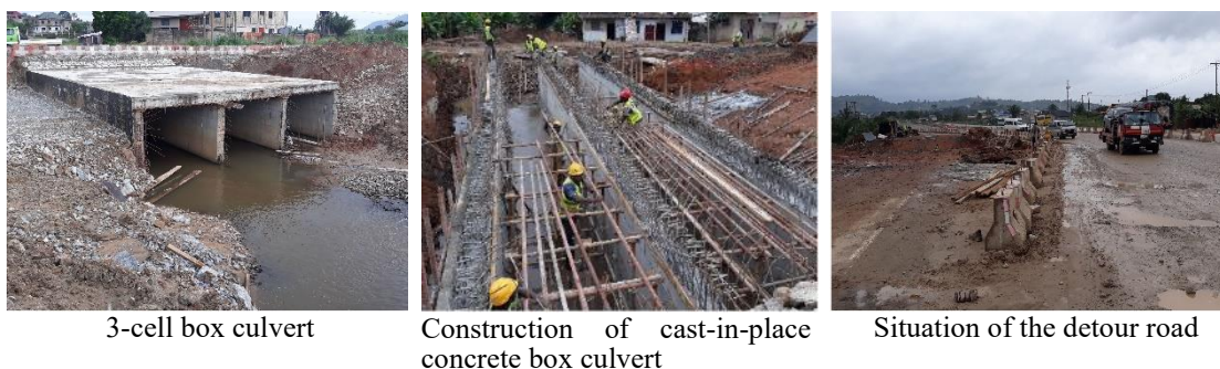
Figure 4-1 Construction Situation of Large-scale Box Culvert by Local Contractors
