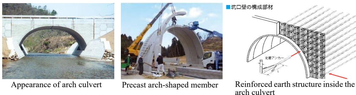
Figure 4-2 Overview of the Arch Culvert Method (TECH SPAN Method)
