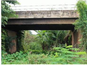
Existing single-span bridge L=13m
