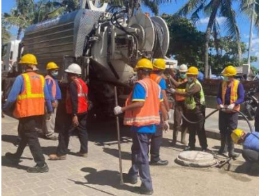
Sewer Cleaning work in Denpasar city
