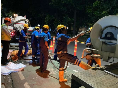
Sewer Cleaning work in Jakarta city
