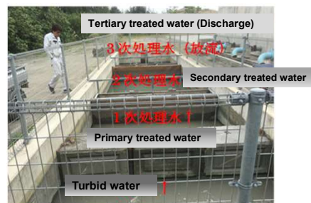
Filtration of turbid water in a gravel extraction site
