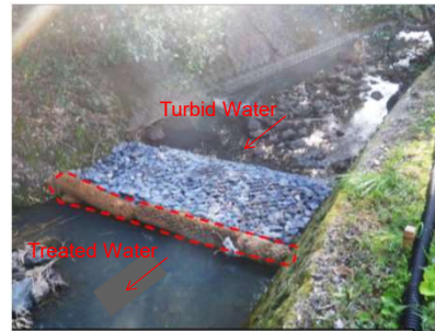
Turbid water treatment with combined use of biolog filter and crushed stones
