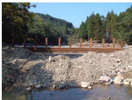
Setting of H beam and biolog filter in mountain streams
