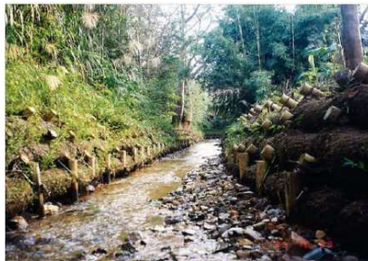
Prevention of small river erosion and conservation/regeneration of vegetation
