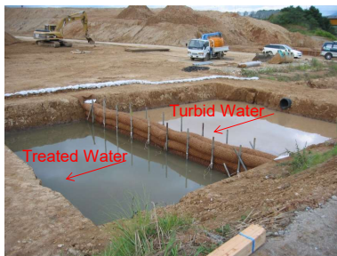
Filtration of turbid water in a construction site
