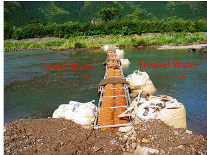
Turbid water treatment with biolog filter alone
