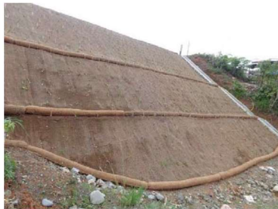
Prevention of road slope erosion and conservation/ regeneration of vegetation
