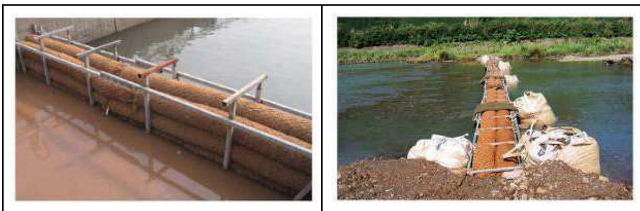
Execution example of the environmentally conscious turbid water filtration for large settling basins
