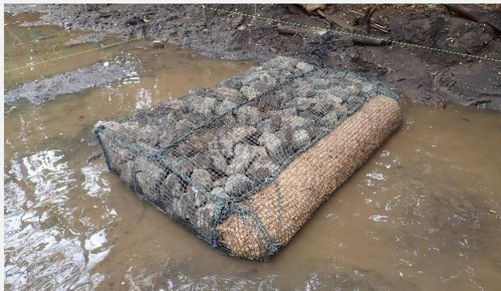
**Photo 3.6 Bio-log Filter unit (Filter unit filtration material with Bio-log Filter)**
