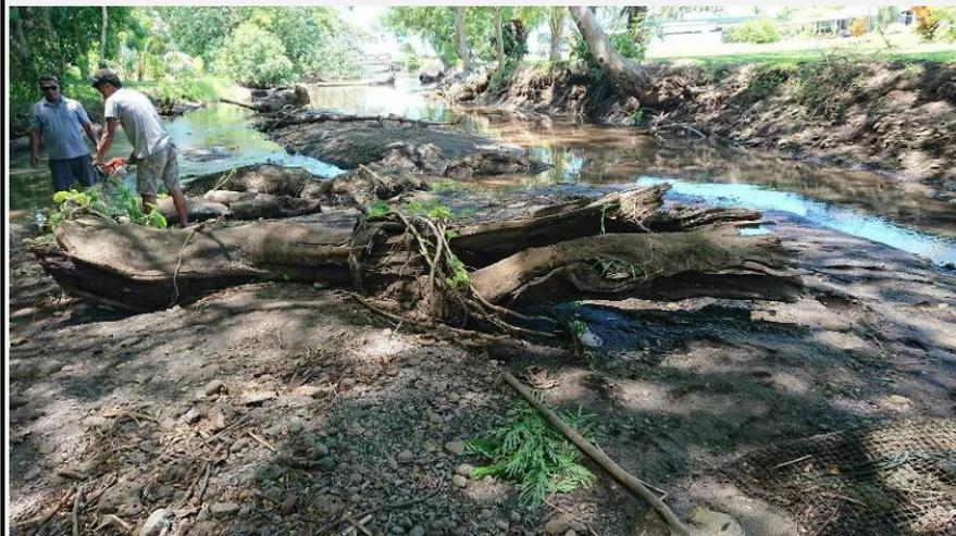
**Photo 3.7 Sediment and driftwood (large trees) captured by the filtration material**
