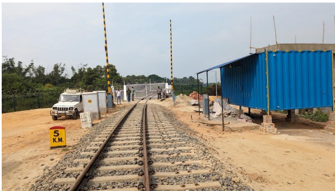
Figure 3-20: Track at the Zero Point (Boundary), Dual Gauge with Readiness for Extra Rail Installation
