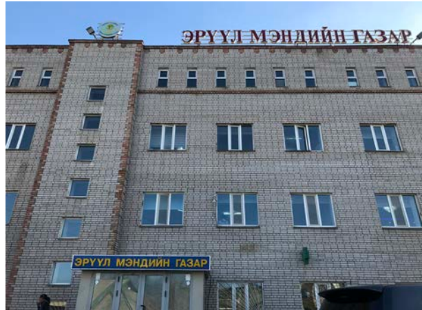
Public Health Center, Darkhan-Uul Province Health Department
