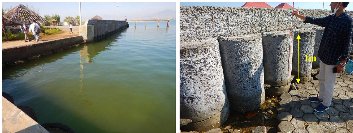
Figure 33 Seawall Condition (Left) and Heightening of Seawall (Right)
