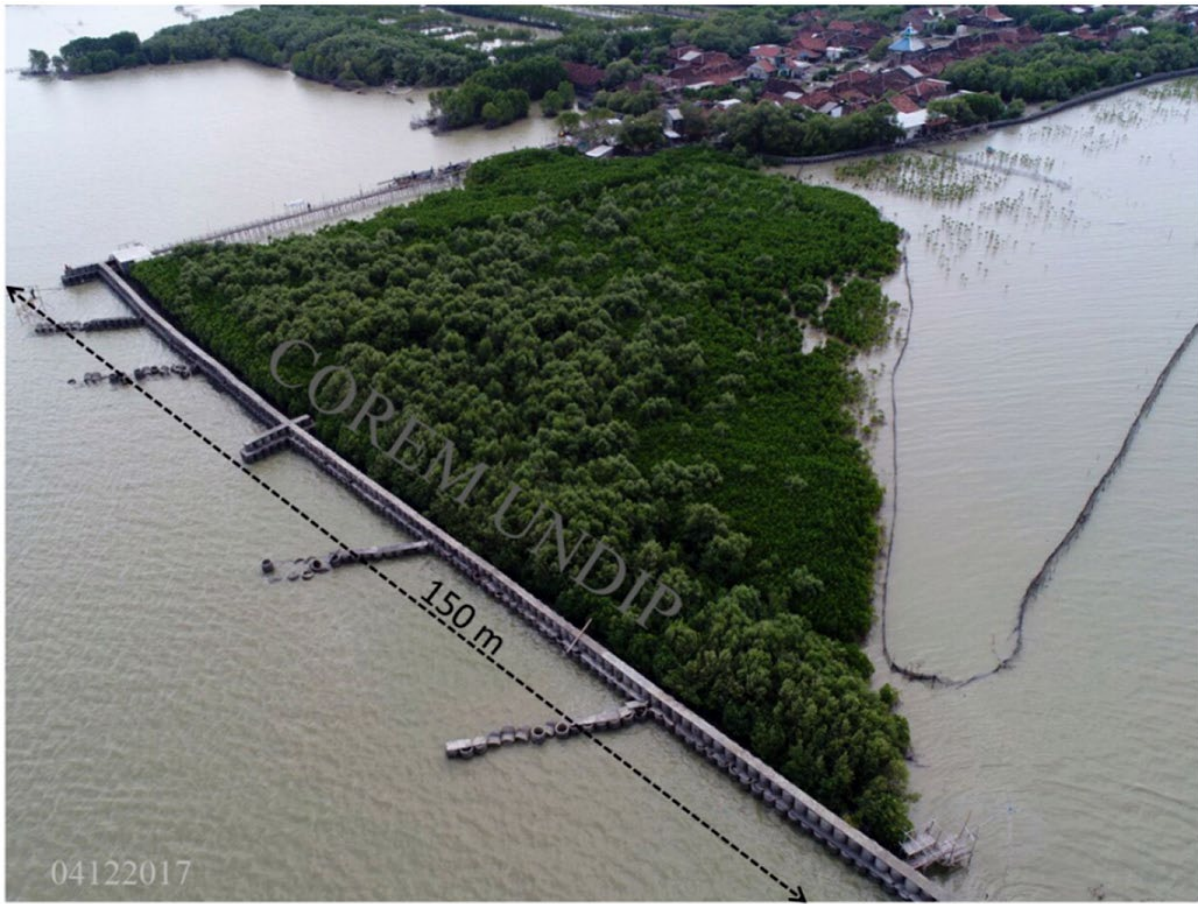
Figure 26 APO (Seawall) Overview
