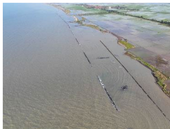
Figure 59 Diffraction wave due to the offshore breakwaters
